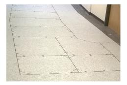
With EJ having the UK's largest range of access covers & drainage gratings we were able to call on the PS4300 recessed duct cover system to provide the solution to meet the contractors' needs. With such a complex cover layout it required all departments to work together from sales, design, production, through to delivery.
